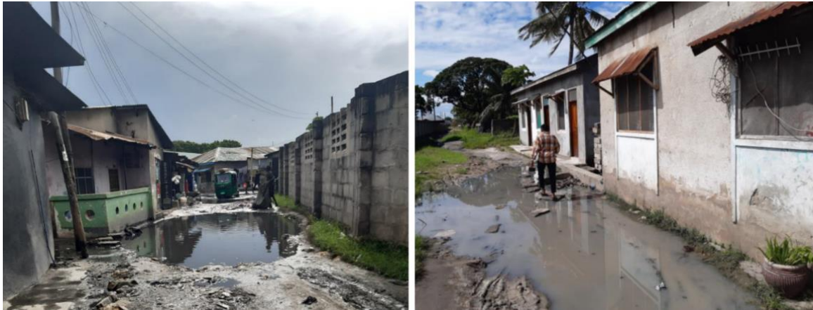
Figure 7: Photos illustrating an example of the environmental hazard on the streets: the formation of rainwater cesspools on the buildings' front veranda. Source: Fieldwork (2022).
