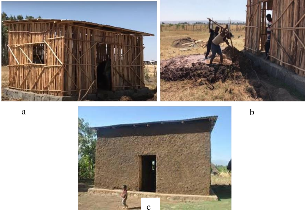
Figure 10: Traditional mud house and its construction process (a) timber frame (top left), (b) mud and straw mixing (top right) (Ralph, 2017), (c) finished mud house or “yechika bet” (bottom).
