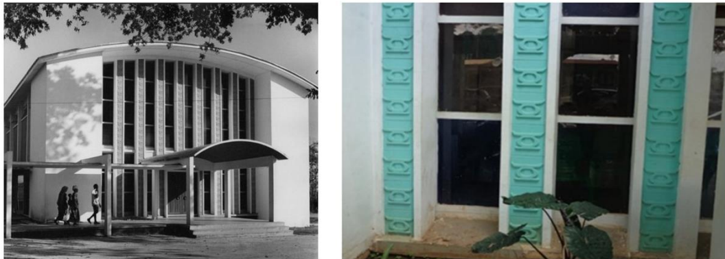
Figure 10: Prempeh Assembly Hall (Adjei and Oppon, 2021).
