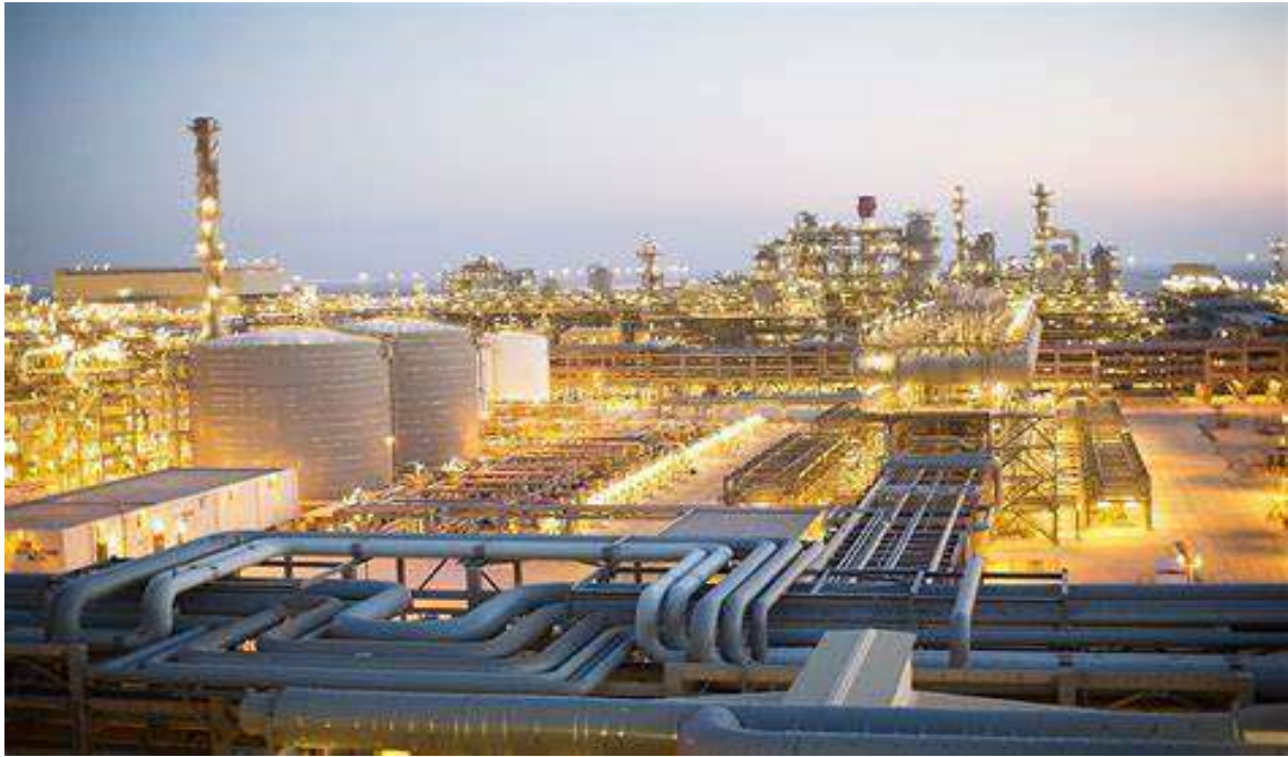
Figure 5: Qatar Pearl GTL Plant (Source: SHELL, 2023)
