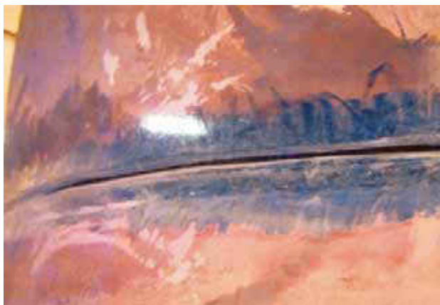
Fig. 11 Repairing of the cracked shell.
