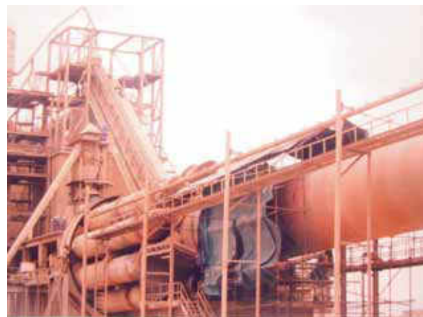
Fig. 7: Typical arrangement of air powered milling machine for turning the rebuilt by welding long shaft with a bearing journal
