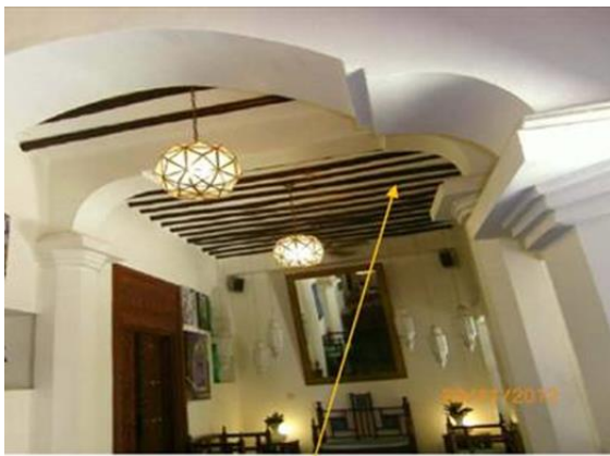
Figure 2: Slab reinforced with mangrove beams.
