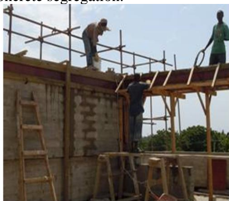
Figure 2: Typical appearance of mortar pan.
