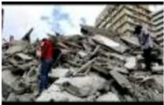
Figure 5: Collapsed building rubbles.
