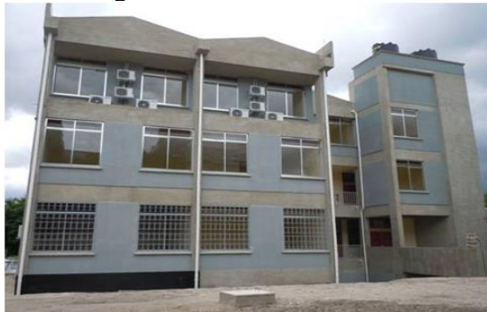
Figure 3: Structure made fro RMC at UDSM.
