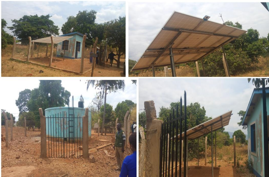
Figure 1: Physical picture for Kikombo water pumping project.
